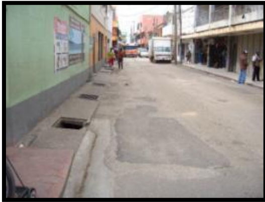
Hazardous Sidewalk in Central Area (could cause serious injury to pedestrians)
