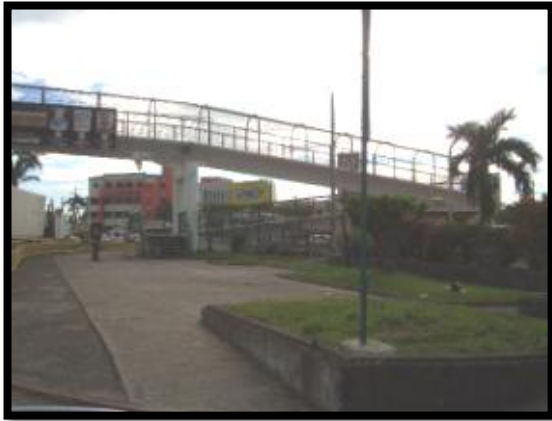
Pedestrian Bridge at Freetown Junction
