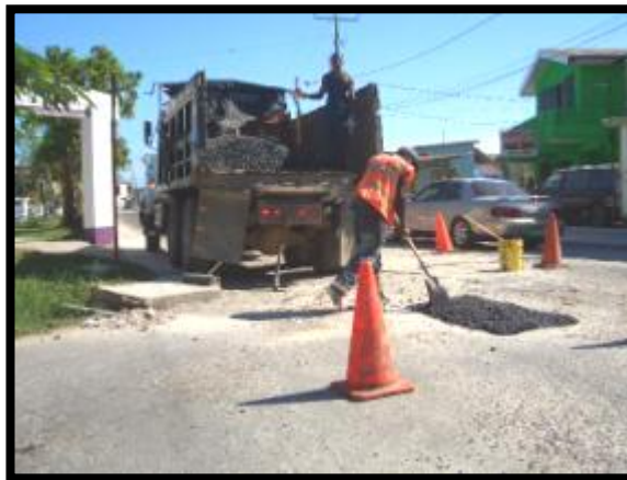
Repair works in central area of Belize City – filling in potholes
