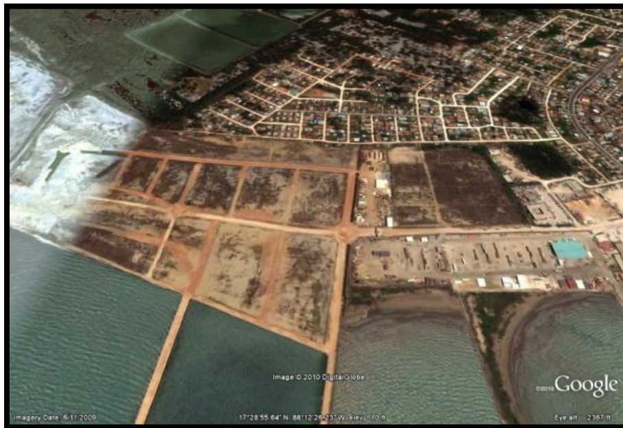
Figure 14: Seaport with On-going Land Filling and Reclamation along Southern Shoreline
