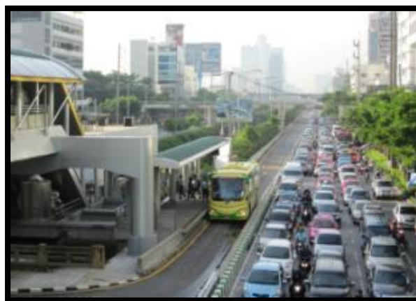
Bangkok BRT Corridor- illustrating the comparative advantage of bus priority measures for road space
